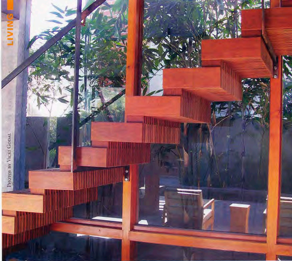
A free-hanging staircase against a glass wall and sliding wood doors adds to the openness of the McKinley home.
