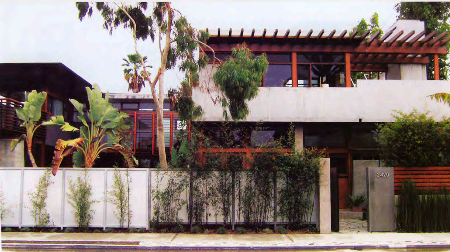
The “green” home of architect David Hertz consists of four buildings on his Venice, Calif., property.
