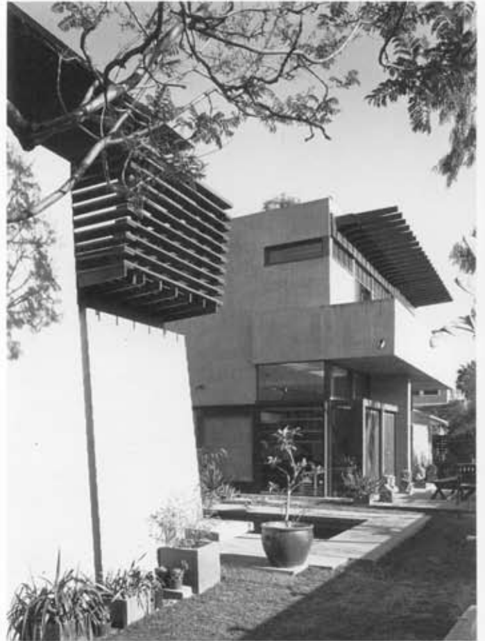
Extension (left) and existing house (right) 増築部 (左) と既存部 (右)
